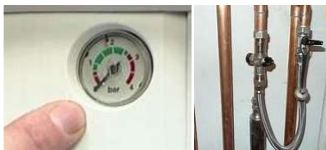
Pressure Gauge (Left) and Filling Loop (Right)
